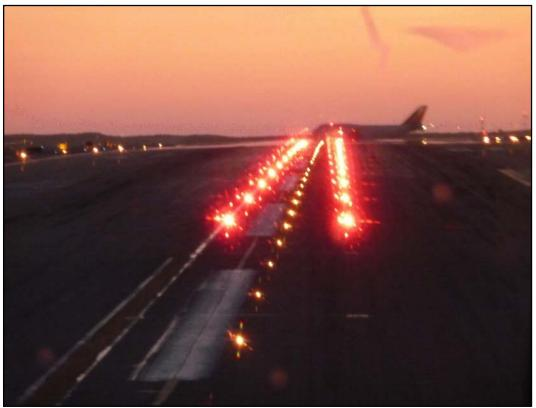
FIG 2-1-14 Taxiway Lead-On Light Configuration
